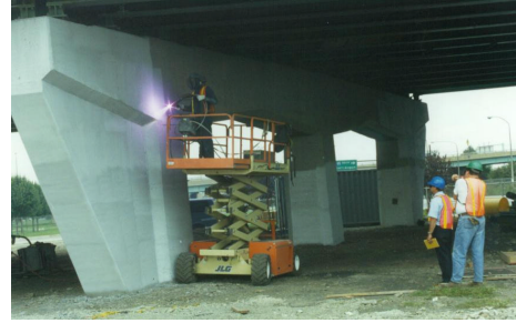
Figure 6. Arc-spray application of sacrificial Aluminum-Zinc-Indium
