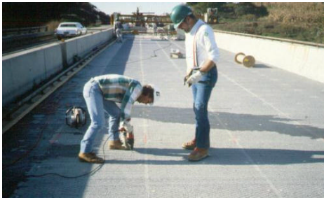
Figure 5. ELGARD Anode Mesh installation on a bridge deck
